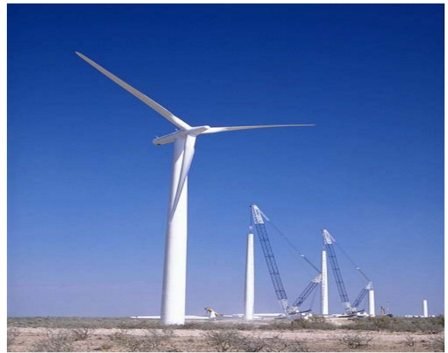
Construction began on these wind turbines at King Mountain Wind Ranch in west central Texas soon after the state passed an RPS in March 1999. The turbines (279MW) began fully operating in December 2001 and provide energy for about 100,000 households a year. Photo by Texas Wind Power Company.
