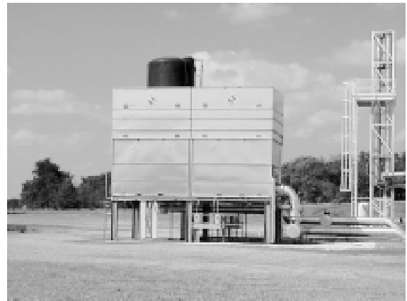
Diesel generator located at the Eagle Mountain International Church outside Fort Worth
