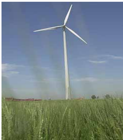
Wind Turbine, Maryland Energy Agency
