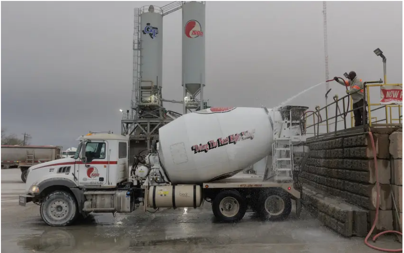
A concrete truck is washed at a concrete batch plant. 📷 Shelby Tauber for The Texas Tribune
