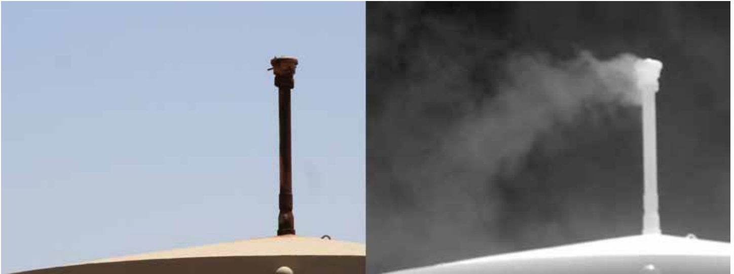
A photo and an infrared image showing emissions from a New Mexico gas compressor station. Photo: Charlie Barrett, Earthworks
