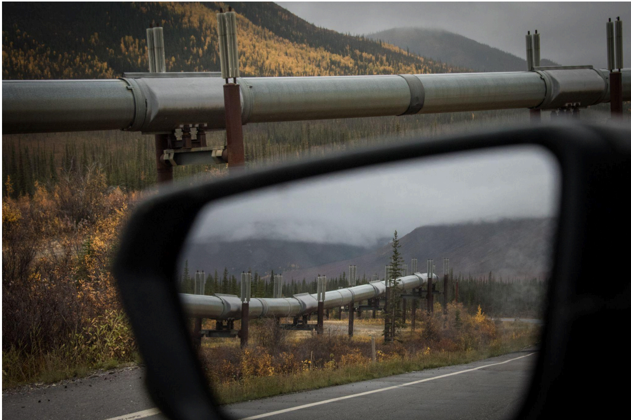
Caption: A photo of the existing Trans-Alaska Pipeline, which carries oil across the state. The proposed LNG gasoline route will partially parallel it. Photo Credit: Lois Parschley
