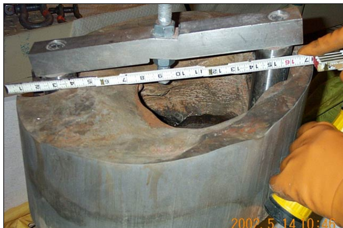
The hole in the reactor head at Davis-Besse, measuring 8" wide.
