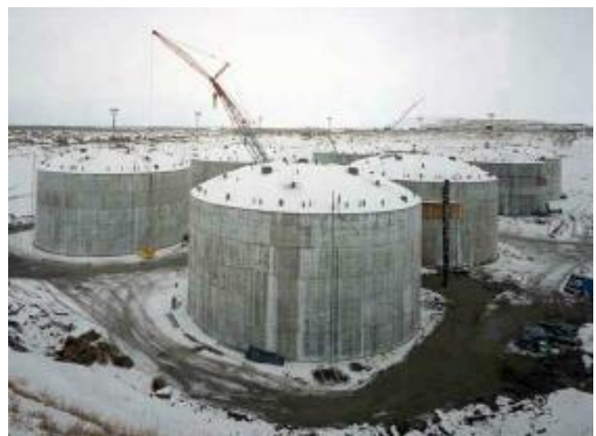
Waste storage drums from reprocessing at Savannah River Site. Photo by the U.S. Department of Energy.
