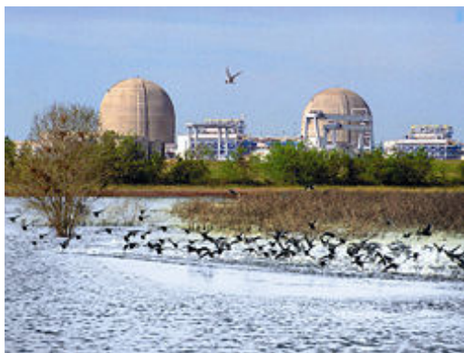
NRC Image of South Texas Project, Units 1 & 2.
