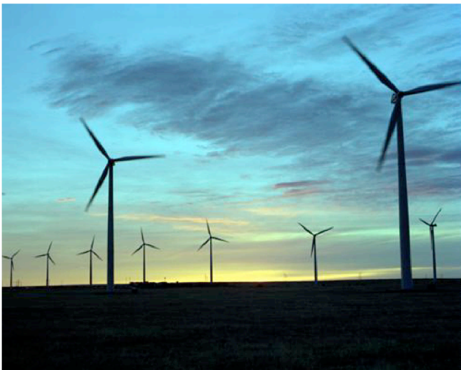
Courtesy: Cielo Wind Power
